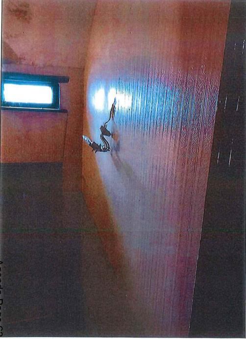
Exposed electrical connection - live status confirmed - Upstairs behind bar
